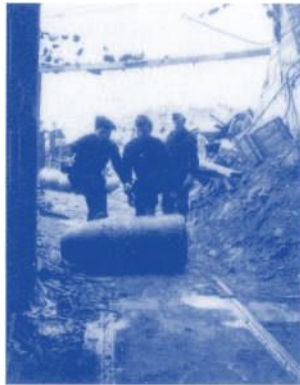
Former German Naval personnel now busy rolling the bombs into the underground tunnels
